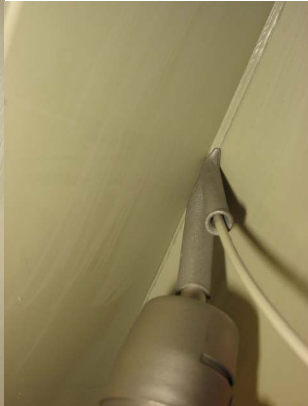
Picture 02: Hot air welding
