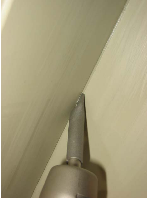
Picture 01: Fixing by a tacking nozzle
